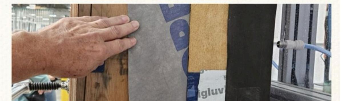
With a team of engineers, Kiwi crew and Shaun St. Amour we came up with a double studded wall system. Where the interior wall is all reclaimed lumber. This sample is pictured where it will eventually land on site, during the deconstruction process.
