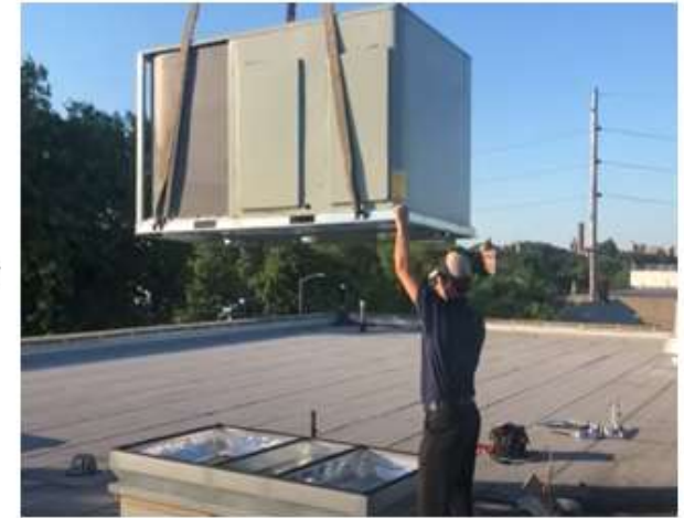
installing new 10-ton unit
