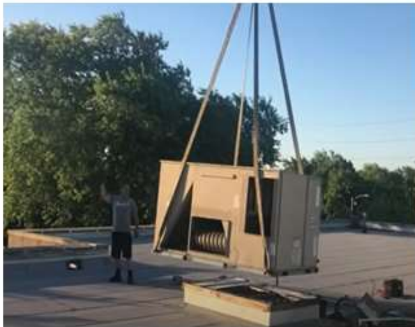
lifting off old 10-ton unit
