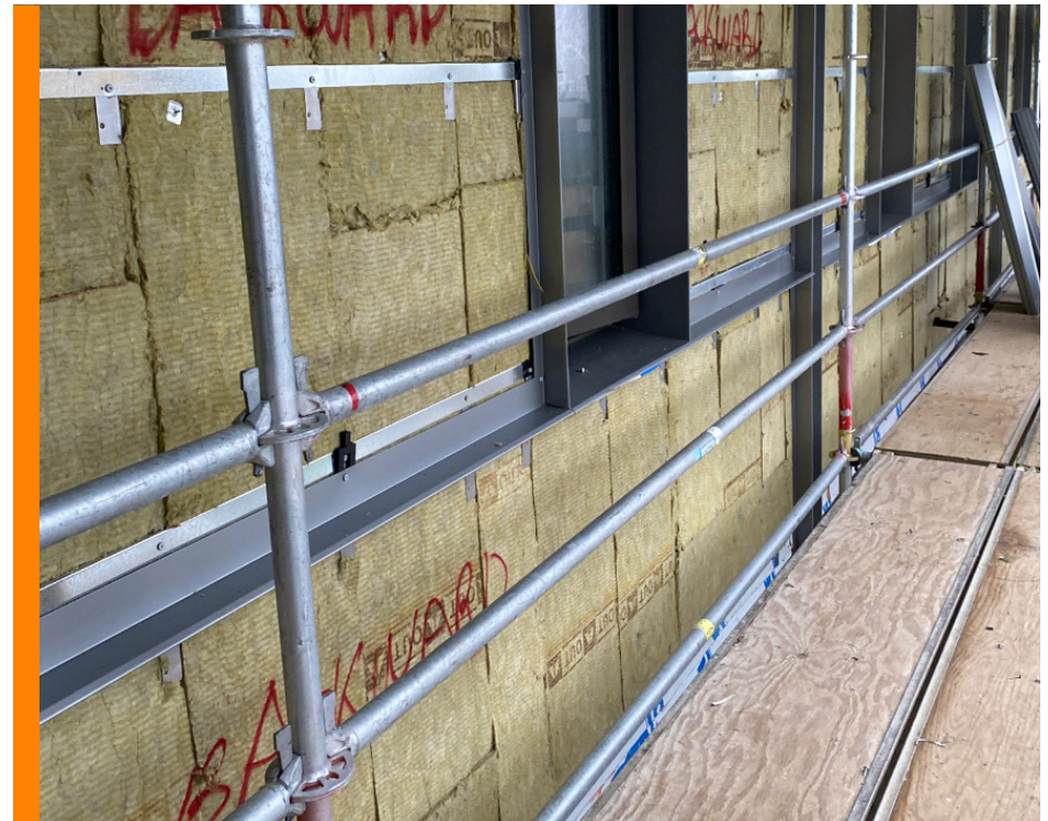
Insulation (Photo credit: Perkins+Will Architects)
