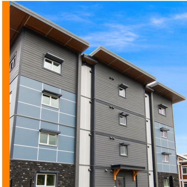
Carrington View Building A (Credit: Skyline Living)
