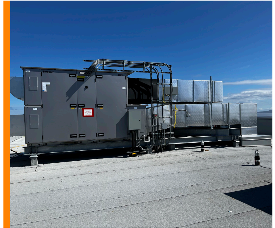
Swegon Gold RX Heat Recovery Ventilator (Photo credit: Introba)
