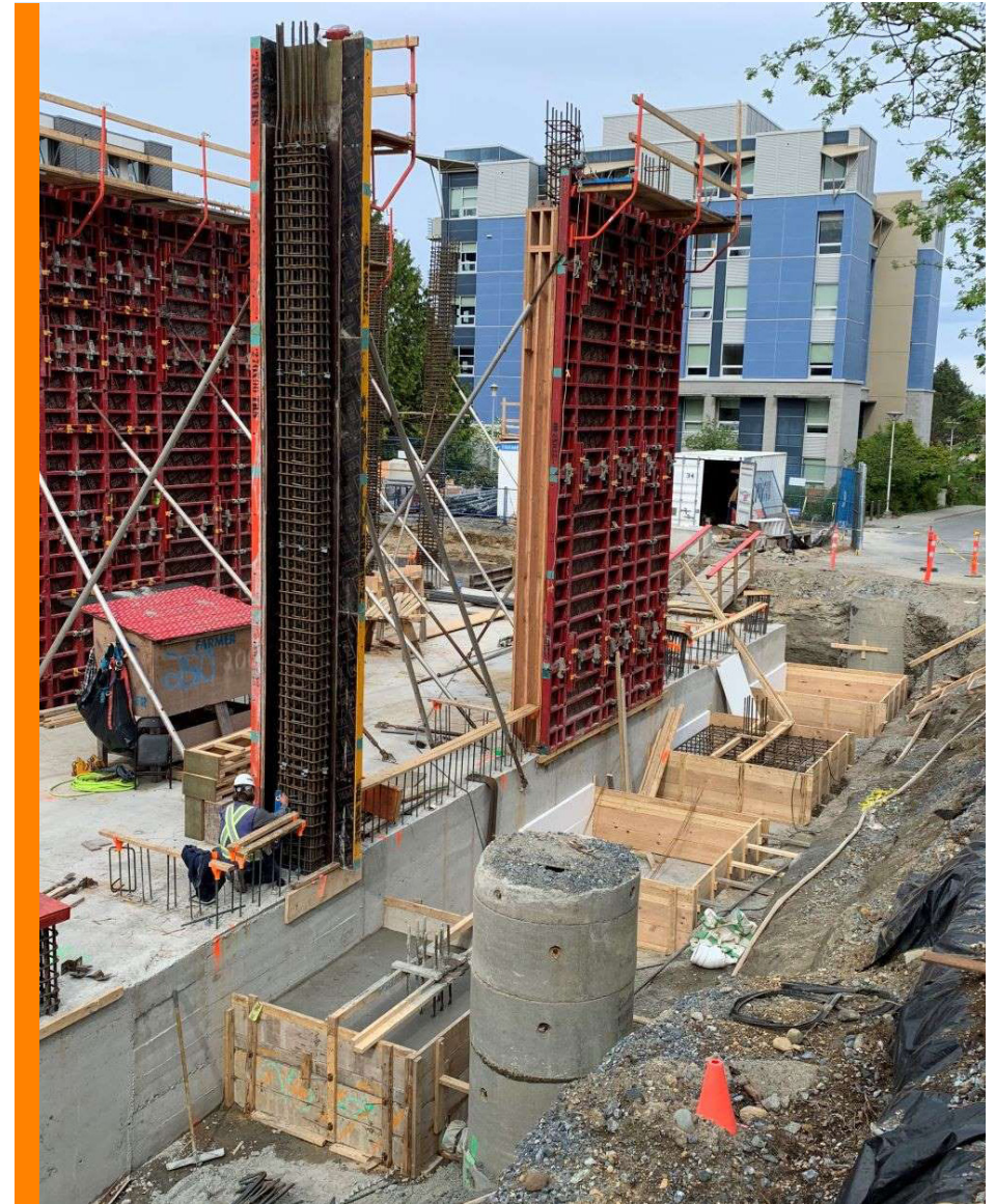
Installation of concrete formwork (Photo credit: Perkins+Will Architects)
