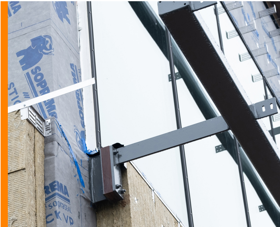
Installation of the sunshades (Photo credit: Perkins+Will Architects)
