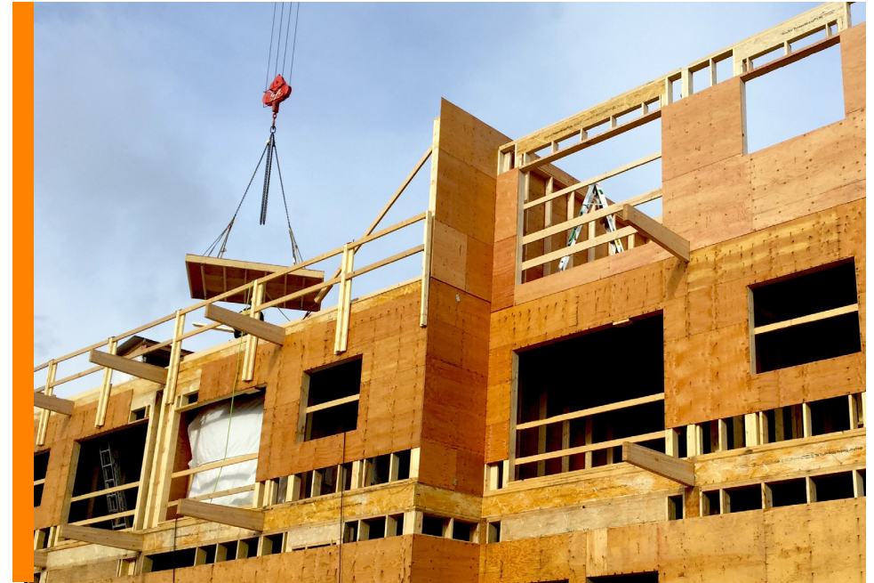
Hoisting of the prefabricated wall panels.
