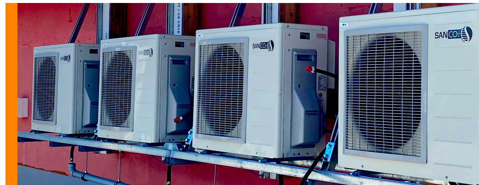
SANCO2 domestic hot water heat pumps.
