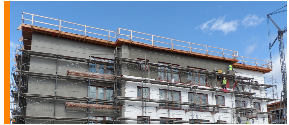
Installation of the EIFS's EPS insulation board.
