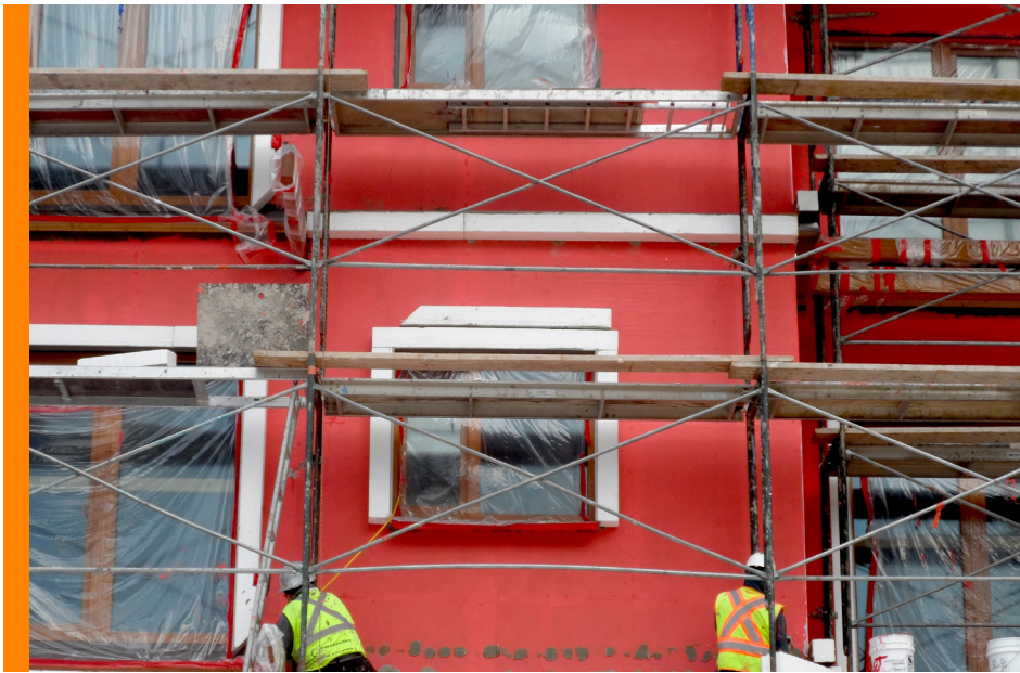
Installation of the EIFS's liquid-applied air and weather-resistive barrier.
