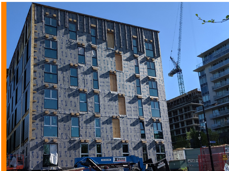
Installation of plywood sheathing and air barrier membrane.
