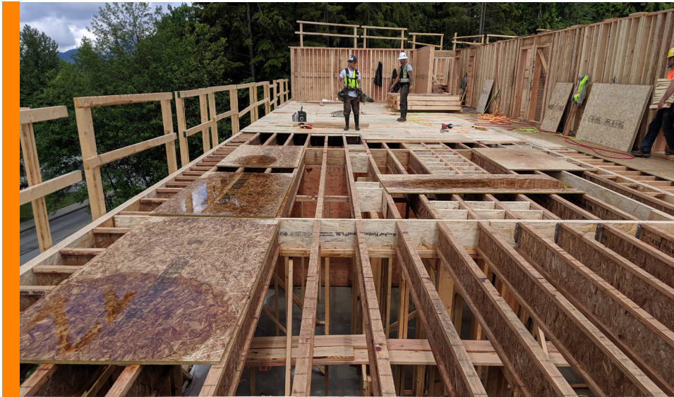
Wood-framed floor structure (Photo credit - Associated Engineering)
