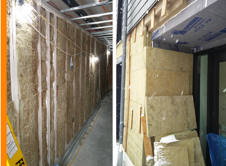
Interior (left) and exterior (right) insulation.
