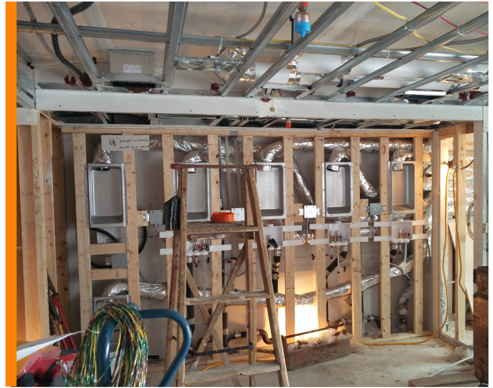
Installation of the ventilation system.
