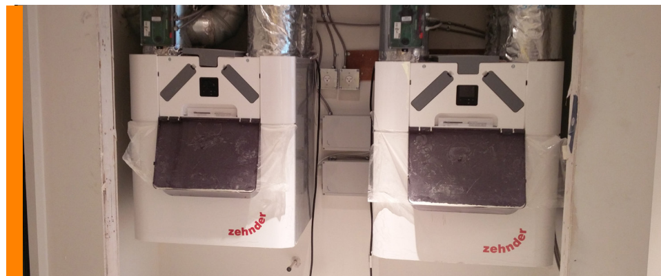
Zehnder heat recovery ventilators.
