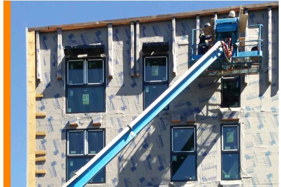
Installation of air barrier over wood block spacers.
