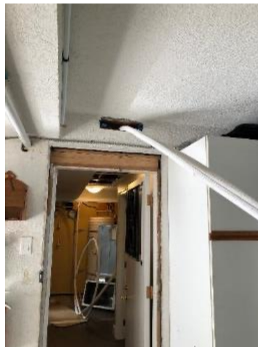
Refrigerant lines – outdoor to indoor
