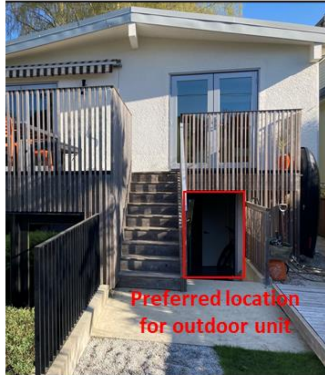
Preferred Location Doesn't Meet Manufacturer Clearances
