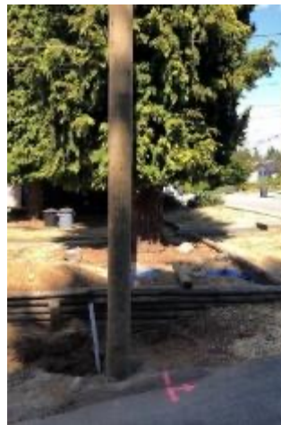
55-year-old Jet fuel pipeline limits pole placement
