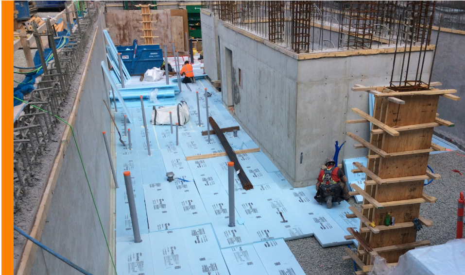
Placement of rigid insulation below the slab-on-grade
