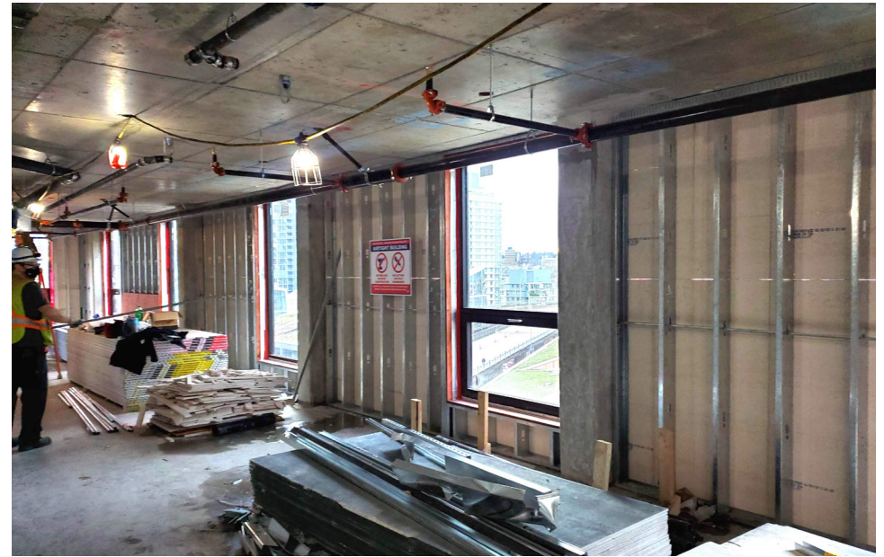
Exterior walls prior to placement of batt insulation
