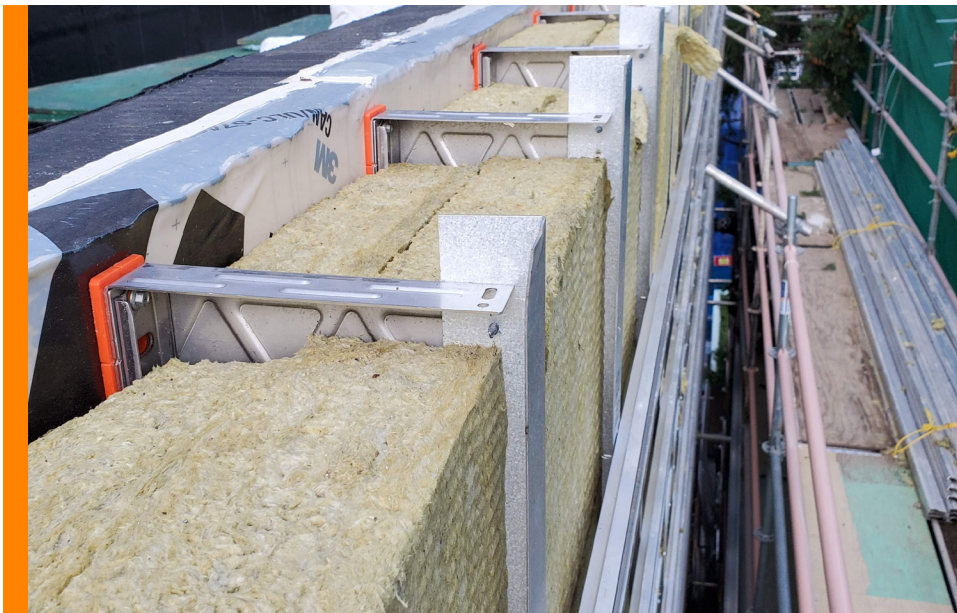
Exterior insulation and cladding attachment system
