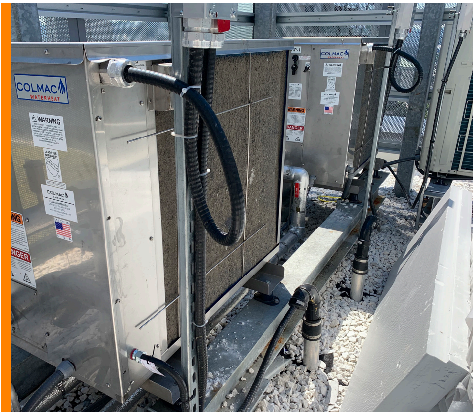
Colmac heat pump water heaters
