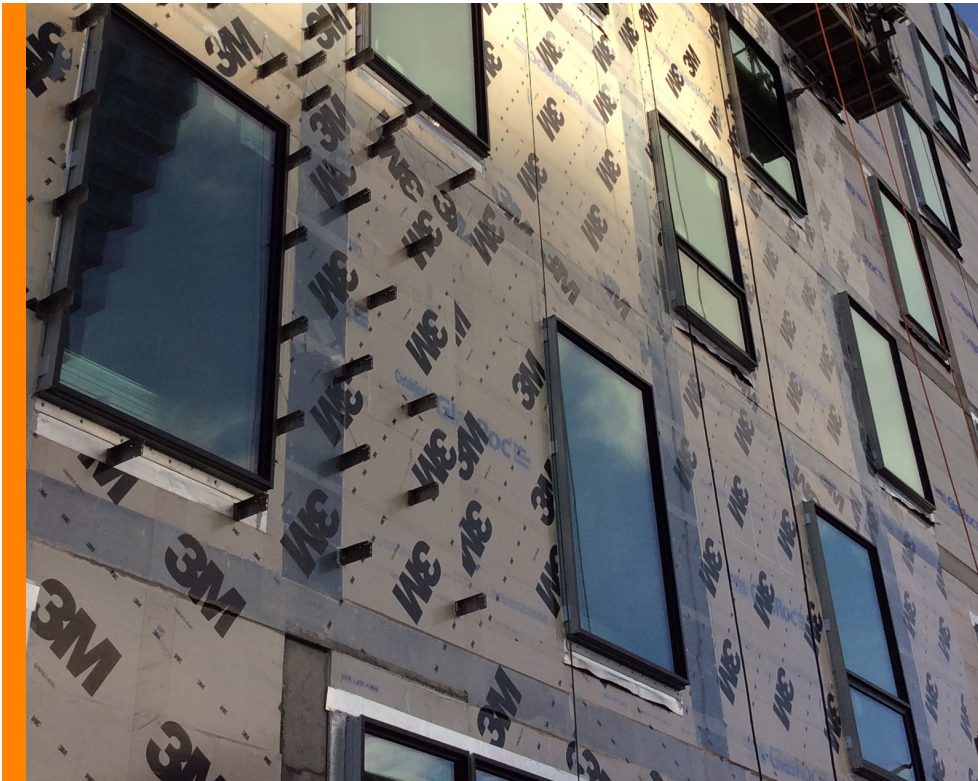
Passive House-certified, triple-glazed, fibreglass-framed windows
