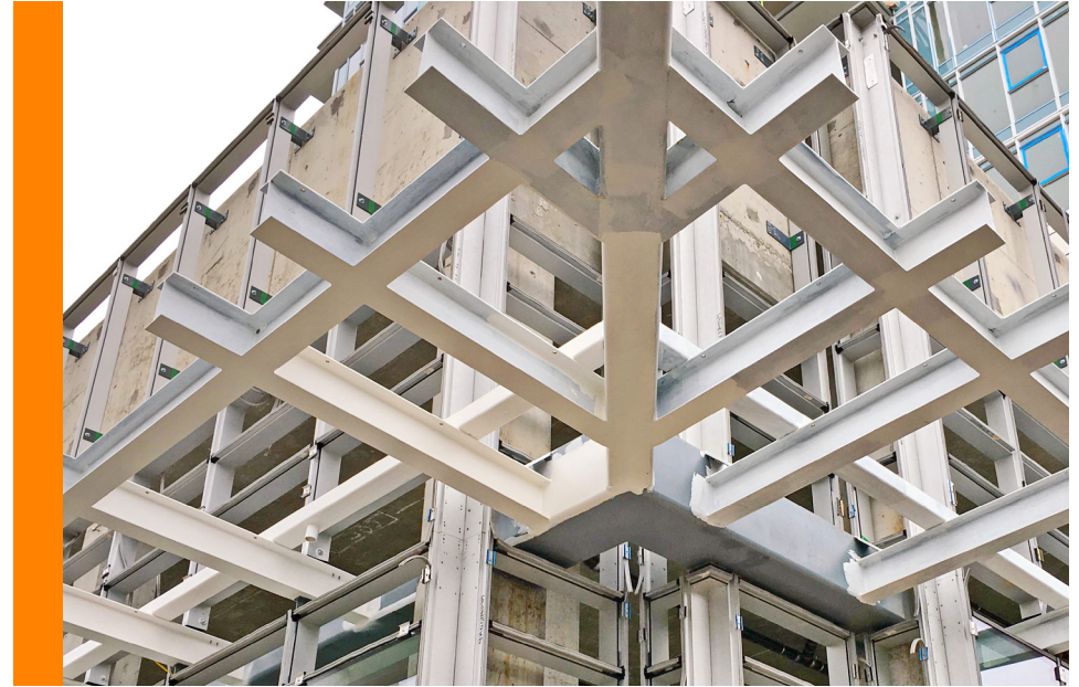
Penetrations through the envelope for canopy supports create thermal bridging
