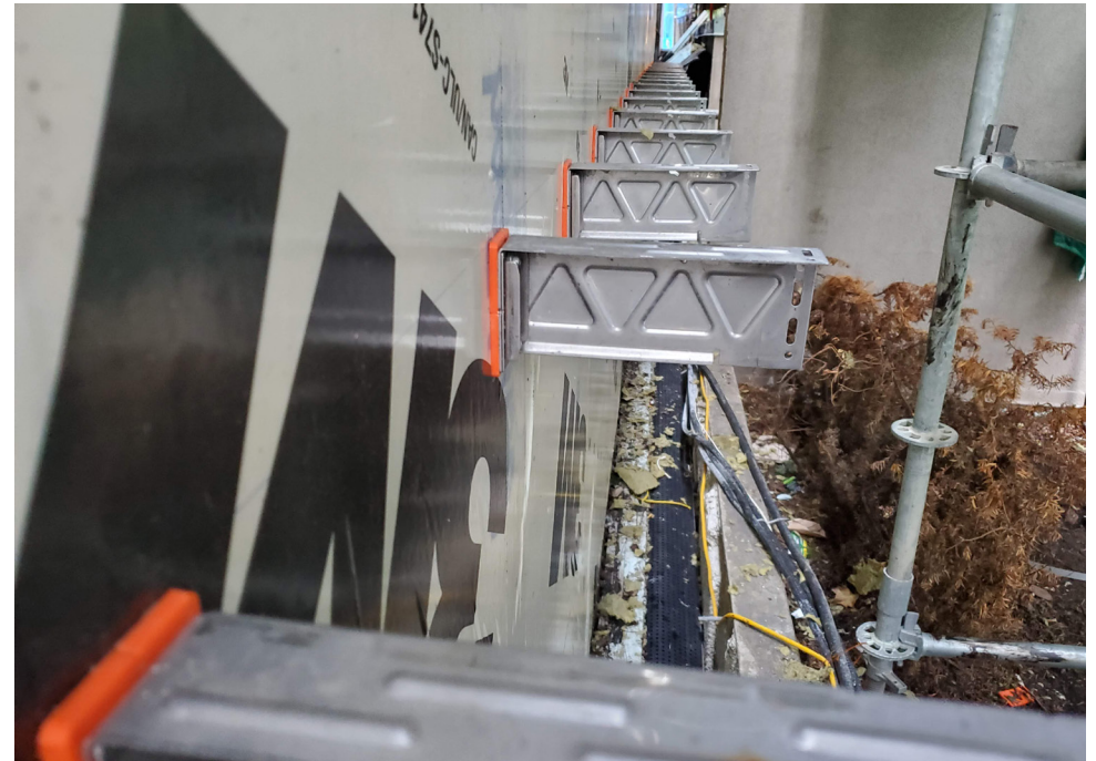
Example Cladding Attachment Arrangement
