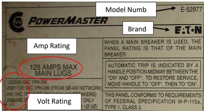
Figure 13. Example of a Subpanel Nameplate
