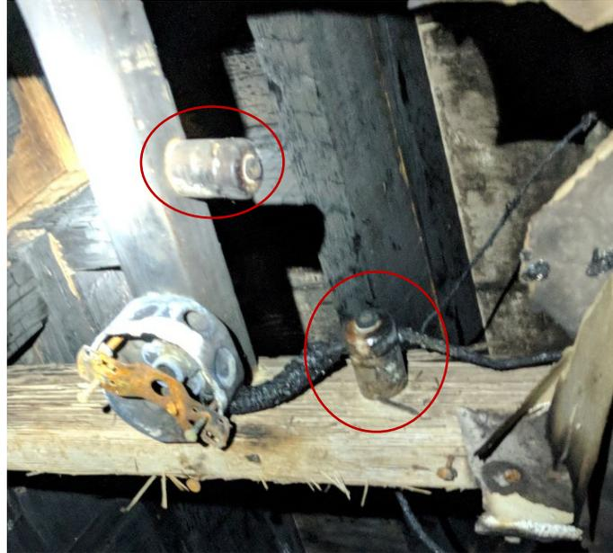
Figure 17. Knob and Tube Wiring
