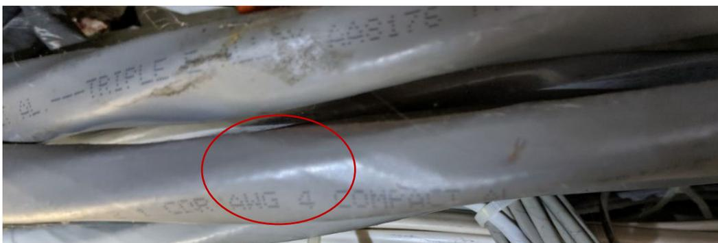
Figure 16. AWG Rating Visible on Exposed Feeder Cables
