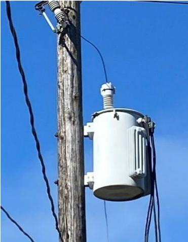
Figure 23. Pole-Mounted Transformer
