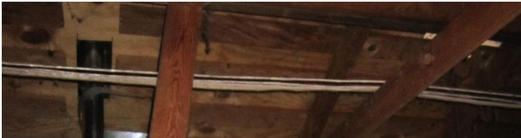
Figure 15. Feeder Cables in an Attic
