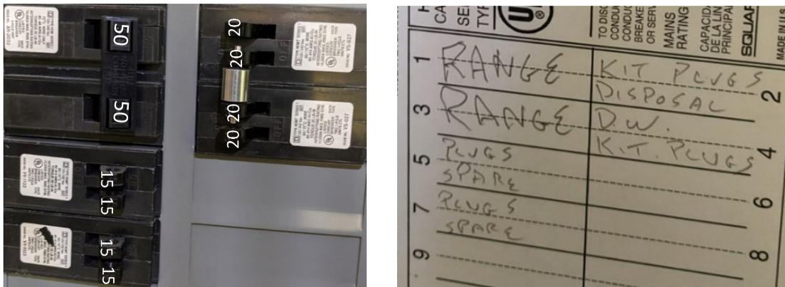
**Figure 10. Subpanel Labeling**
