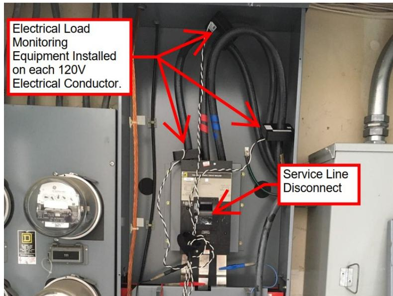
**Figure 26. Load Monitoring Equipment**
