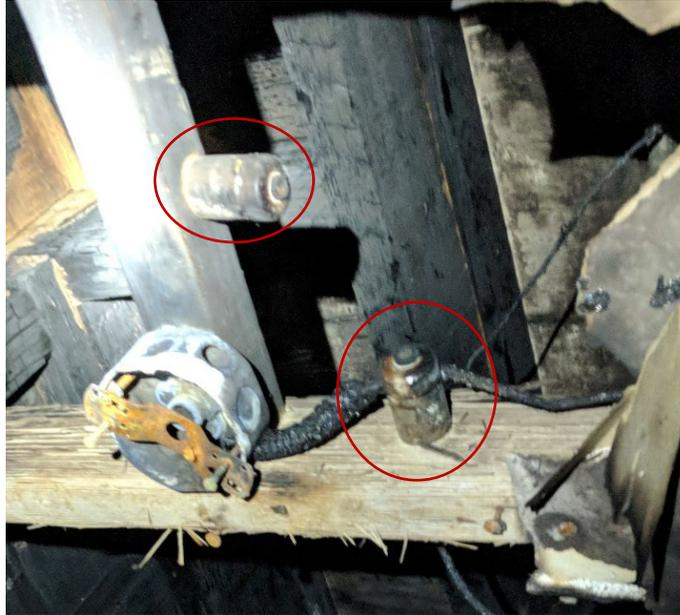
Figure 17. Knob and Tube Wiring
