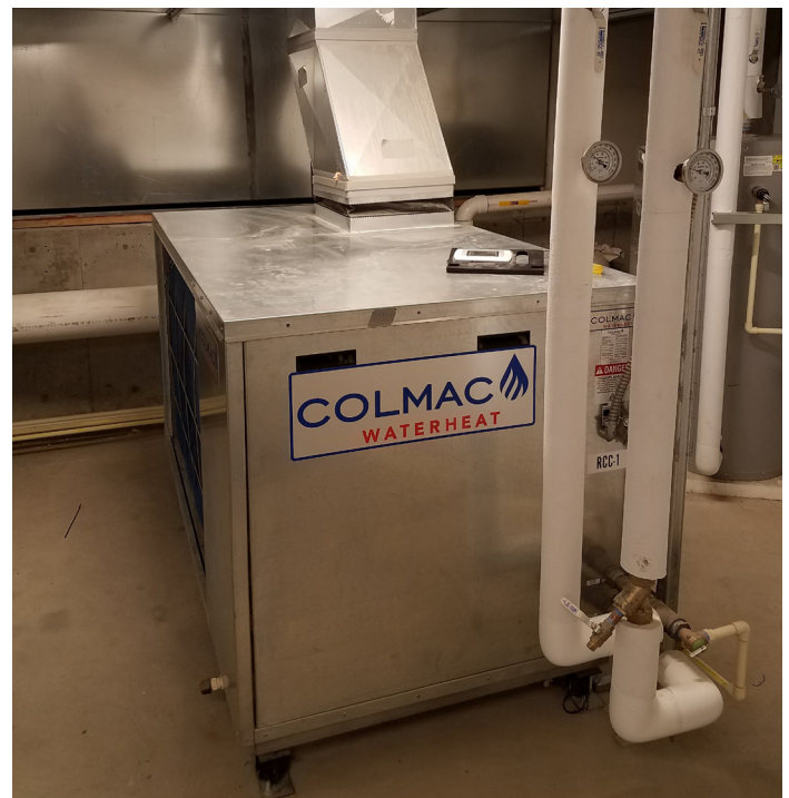
Colmac heat pump located in the parkade floor (Credit: Ecotope Inc.)
