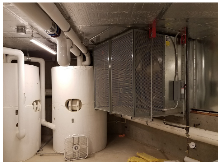
Indoor primary storage tanks in the mechanical room (Credit: Ecotope Inc.)
