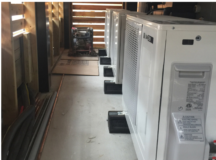
The outdoor units of a heat pump in a high-performance townhouse in Vancouver, B.C. (Credit: Futrhaus, b Squared Architecture Inc.)
