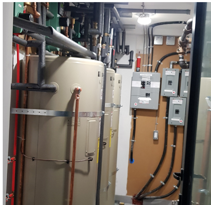
Hot water tanks of Sanden CO 2 heat pumps in a high-performance townhouse in Vancouver (credit: Futrhaus by b Squared Architecture Inc.)
