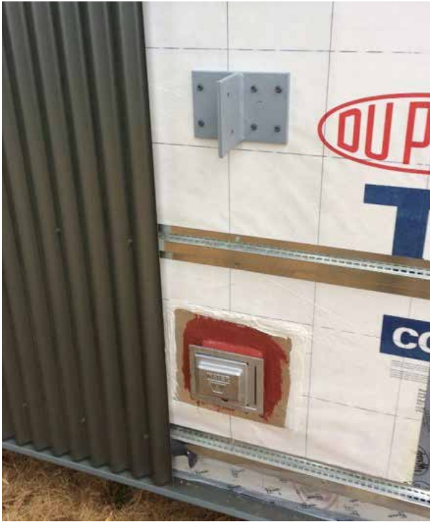
Mock-ups of various wall penetrations
