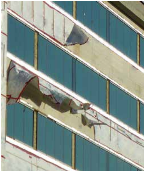
Damaged air barrier during construction
